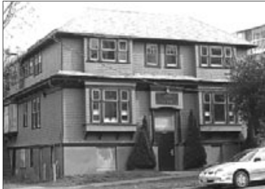
1176 Yates Street - Boarded up in November 2003. Approved for 17 housekeeping units.
