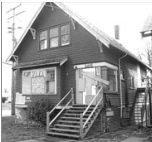
2415 Quadra Street - Derelict and then fire damaged. Now up for sale.
