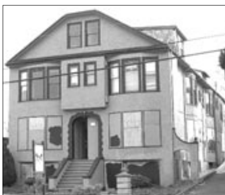
2321 Cook: Boarded up in Sept. 2005: approved for seven suites and seven housekeeping rooms
